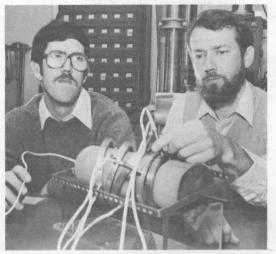
ANELASTIC STRAIN RECOVERY technique is possible because of this patented tool designed by David Holcomb (right) and Mike McNamee (both 6232). It can detect core movements (strain relaxations) as small as one-millionth of an inch.
